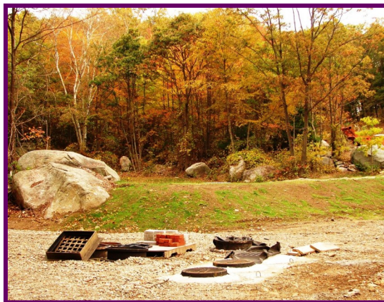
Storm drains and sewer pipes have been installed (below).
